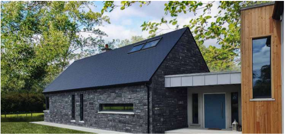
Glenmore Limestone Dry Build
