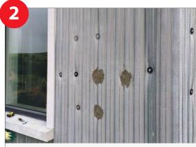
Ribbed galvanised expanded metal is fixed to the wall. This provides a suitable surface for adhesion.
