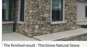
cladding fixed on to external insulation.
