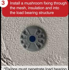
\*Fixings must penetrate load bearing structure to a min. depth of 50 mm.
