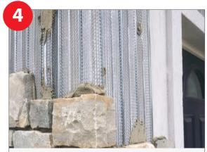
Large galvanized washers are used with the fixings. Fixings are also countersunk in to the insulation/mesh. Use approx 15 - 20 fixings per sheet of mesh.
