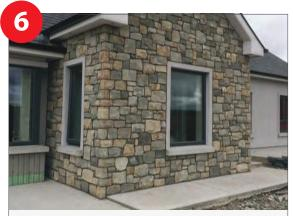
The finished result - ThinStone Natural Stone cladding fixed on to external insulation.
