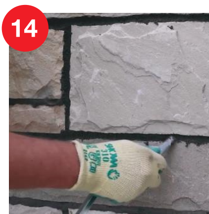
14 Rake pointing mortar when just dry, but not hard.
