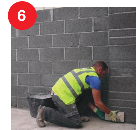
Apply the stone, starting at a corner
