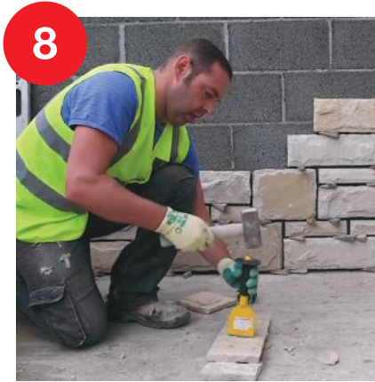
8 Cut stone as needed. Use bolster chisel or a small grinder
