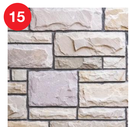
15 Finished wall. All Done!
