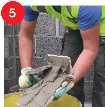
Apply adhesive to back of stone
