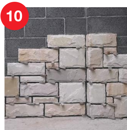
10 Allow 8 hours drying time for adhesive
