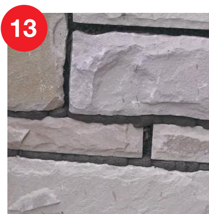
13 Allow pointing to dry (2 to 4 Hours)
