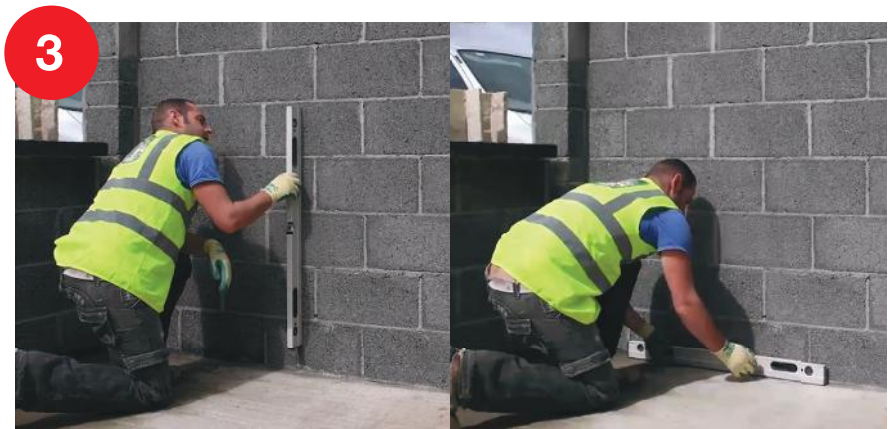
3 Check wall alignment, both vertical and horizontal
