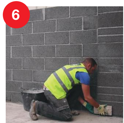
6 Apply the stone, starting at a corner
