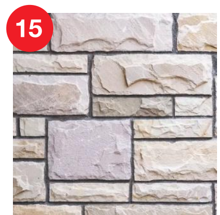
15 Finished wall. All Done!
